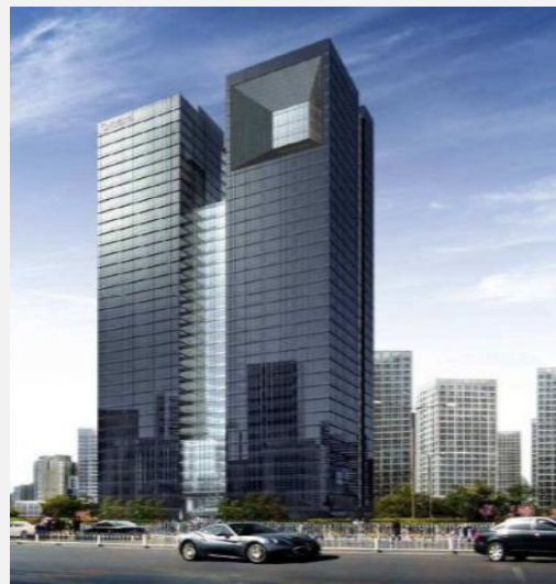
IFC Tower 16 th - 17 th Floor
